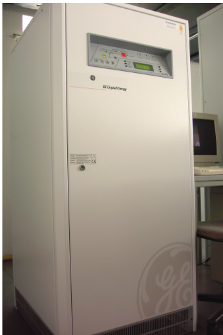
Zentrale USV General Electric SP40
